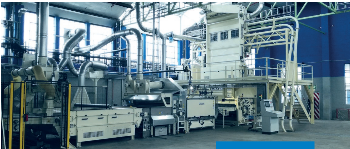
Airlay resinfelt line in operation
